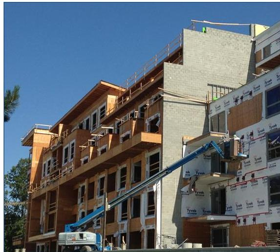
Figure 1: Typical masonry wall in wood frame construction.
