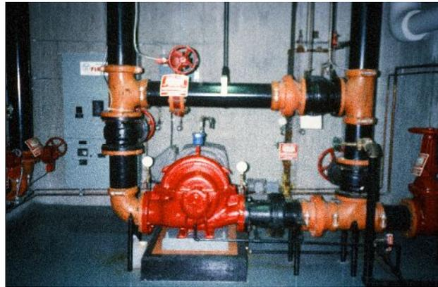
**Figure 12: Booster pump (electric drive)**
