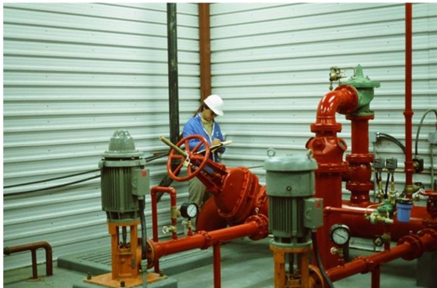
Figure 1: Typical fire pump arrangement taking suction from reservoirs.
