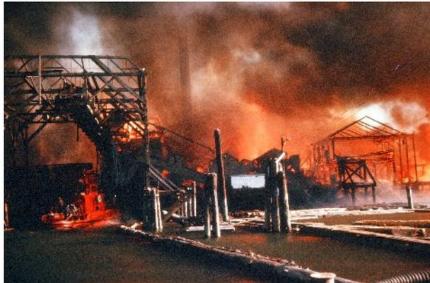
Figure 11: Lack of sprinklers in one area led to this conflagration/total loss of a fully sprinklered building.
