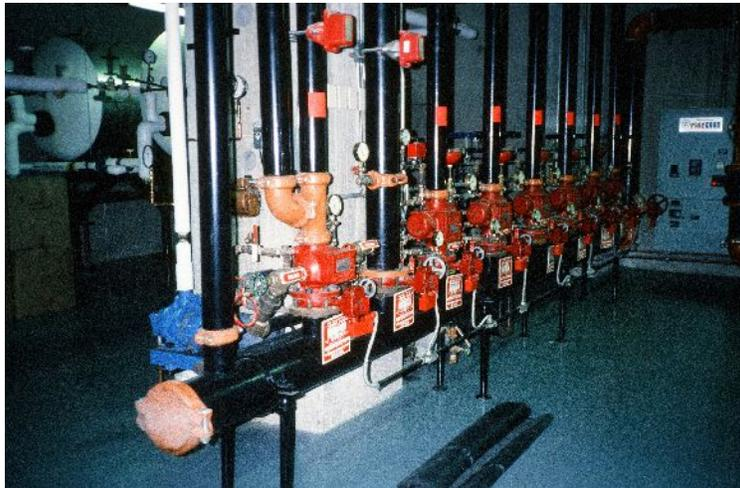
**Figure 9: Sprinkler system manifold for a large facility.**
