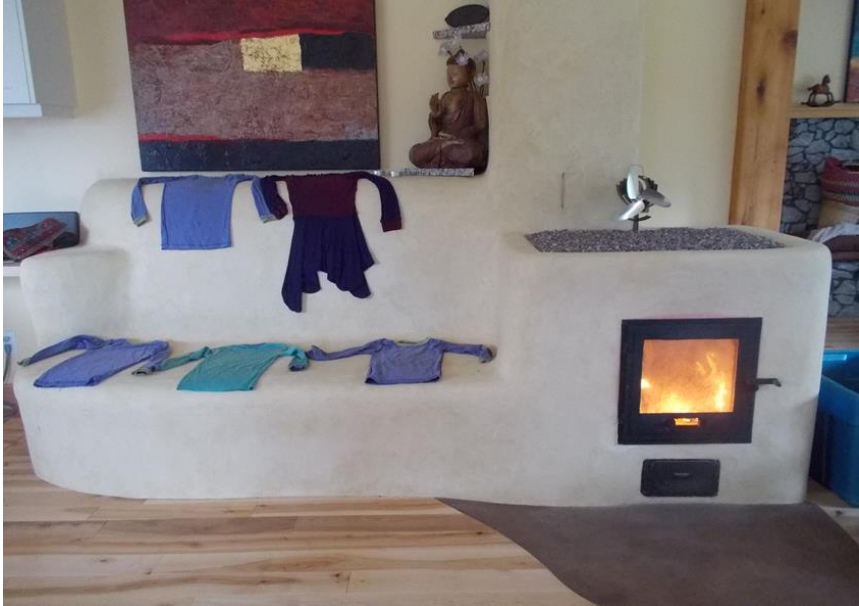
Figure 10: Cob-skinned Grundofen with heated bench and backrest.
