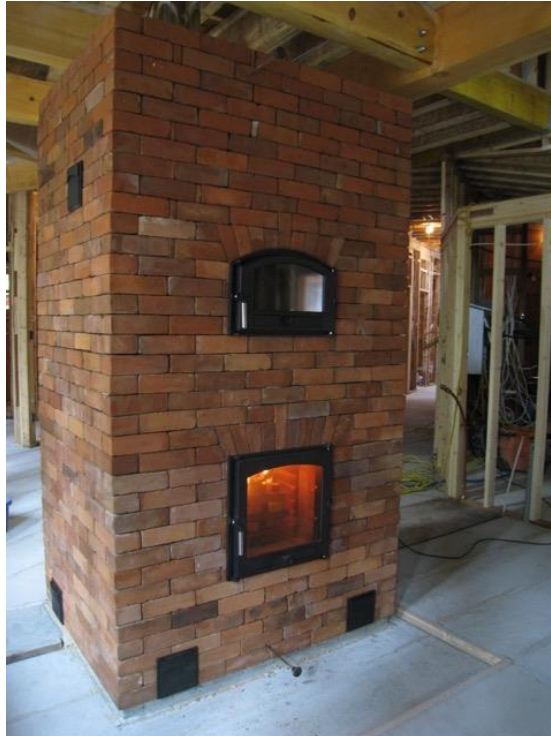
Figure 1: Typical Contraflow Masonry Heater being fired (test phase only-hearth not completed)
