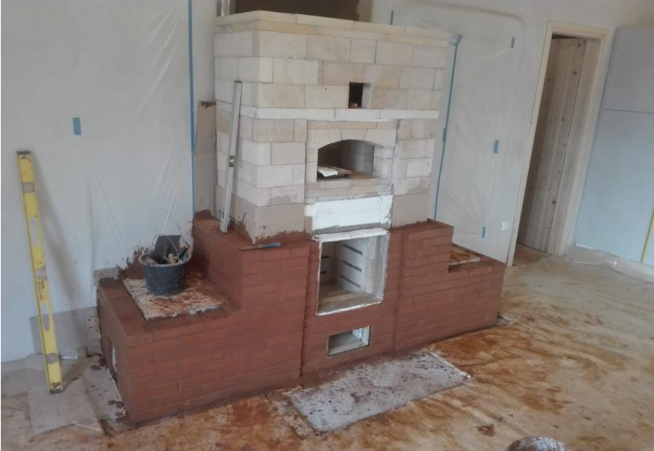
Figure 8: The 'Core' of the heater constructed of firebrick and refractory mortar is separated from the 'Skin' of the heater by cardboard and ceramic fibre.
