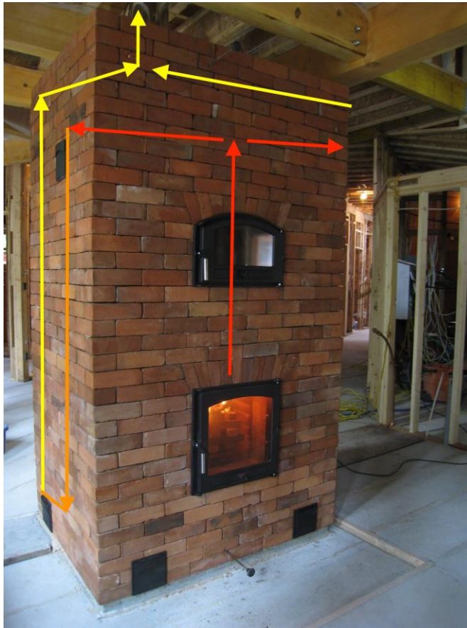
Figure 6: Superimposed arrows showing flow direction on an actual unit.
